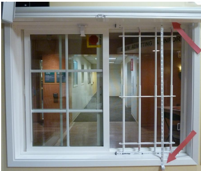
You can also measure and install the guards on the outside of the window casing as shown above.
