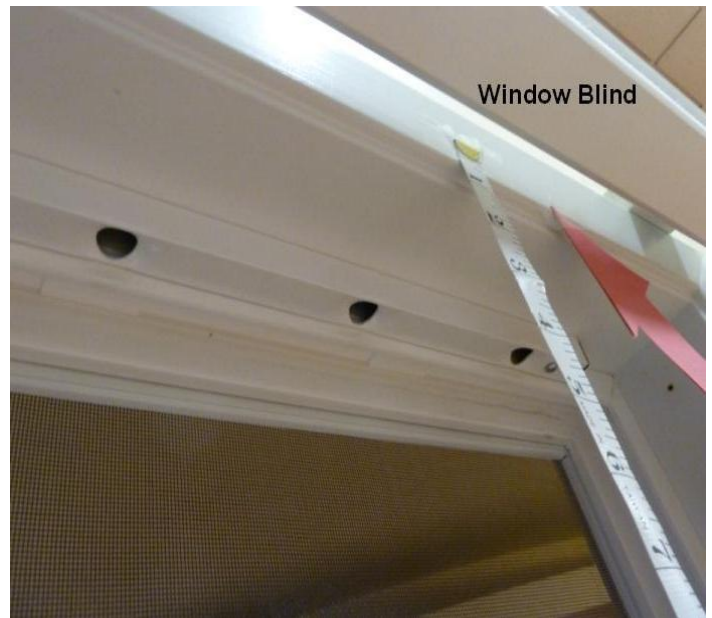
Consider your window treatments when determining placement. Photo shows a close up of the top of the window. Guard is mounted inside, close to window; blind is installed on the outside casing.
