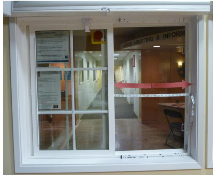
With window open: Measure window opening from inside jamb, right to left. (Usually screened area)
