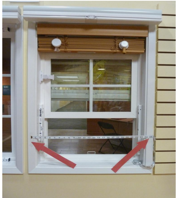
You can also measure and install the guards on the outside of the window (casing) frame as shown.
