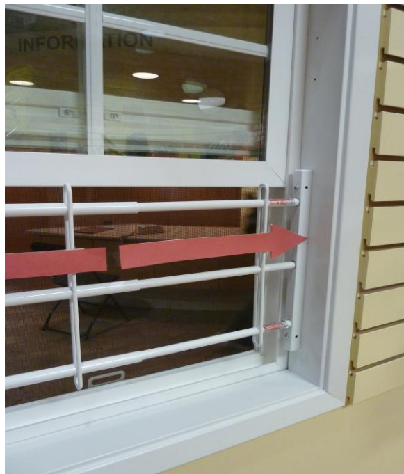
Close up of typical installation on inside of window frame.
