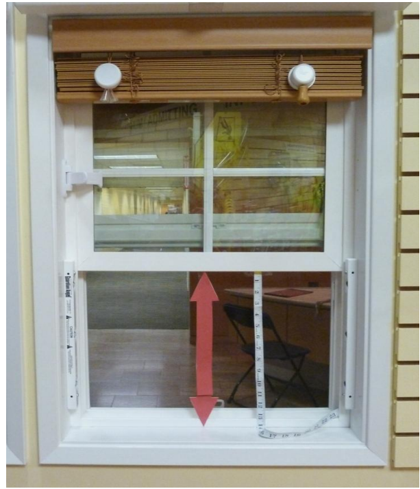
With window open: Measure from windowsill to top of window opening. (Usually screened area)
