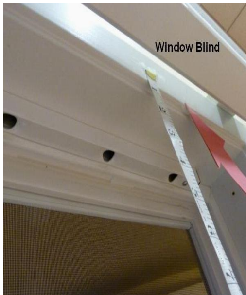
Photo shows a close up of the top of the window. Guard is mounted inside, close to window; blind is installed on the outside casing.
