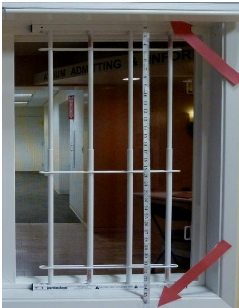
You can measure and install the guards on the outside of the window casing as shown above.
